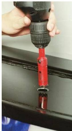
Figure 5-2: Drilling the antenna hole
